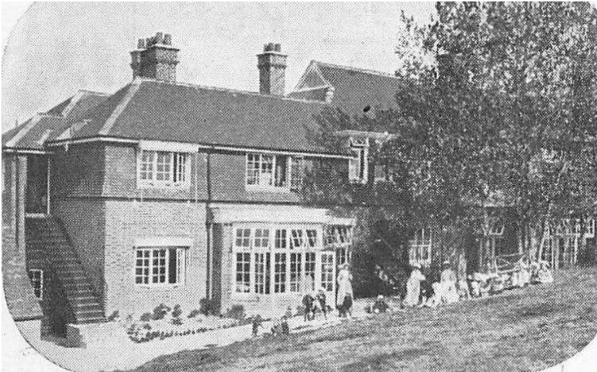
Figure 4. The Home at Bexhill-on-Sea
