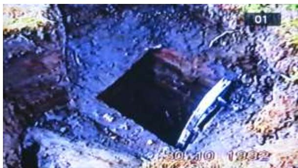
Figure 24. Entrance to tunnels
