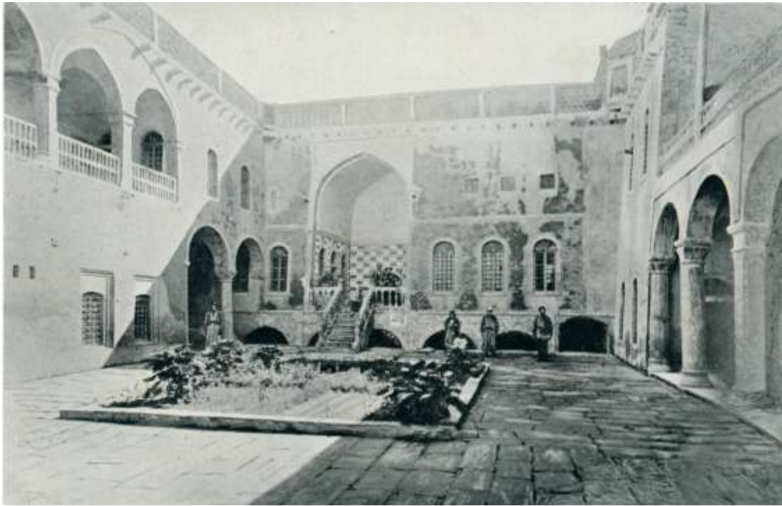
House in Mosul
