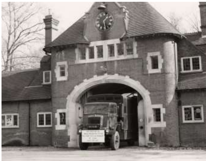
Figure 34. Coach-house with 1943 Bedford QL lorry
