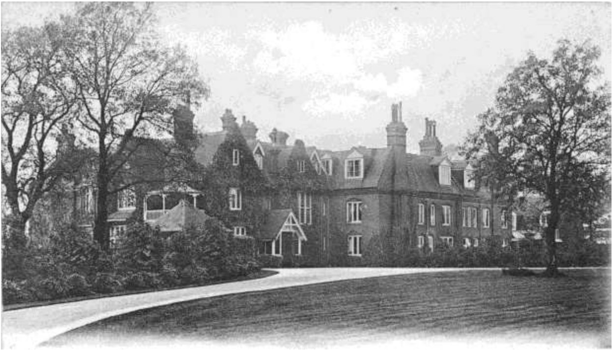
Figure 14. Broadoaks prior to addition of the east and south extensions
